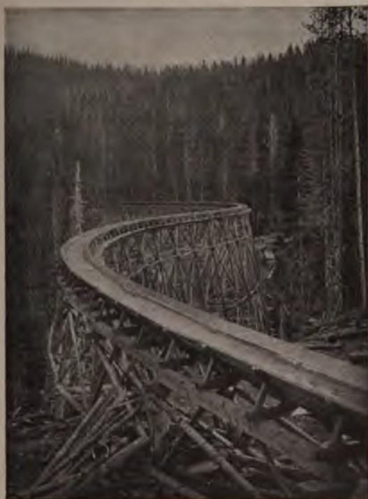
FIG. 124.—A V-Flume for transporting Mining Stulls. Montana.
